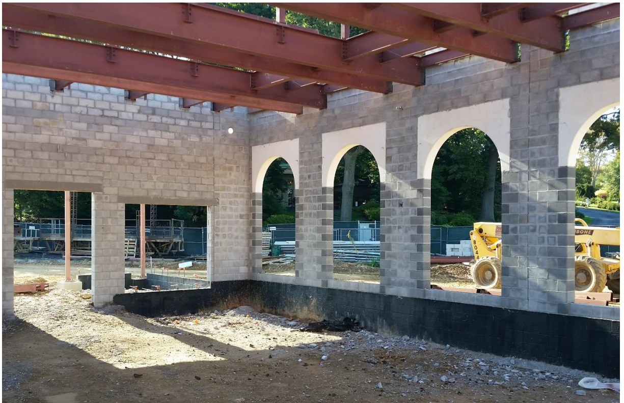
Reinforced masonry shear walls with under construction. (photograph © Keast & Hood)
