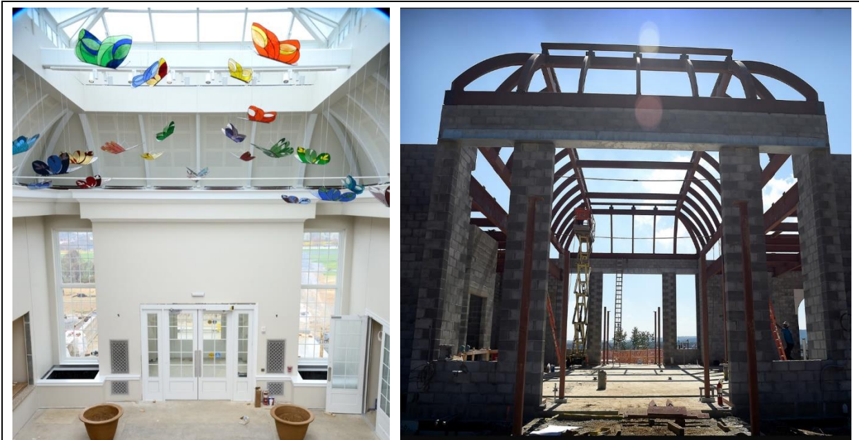
In construction view of the architecturally exposed curved steel framing for the atrium. (construction photographs © Keast & Hood)
